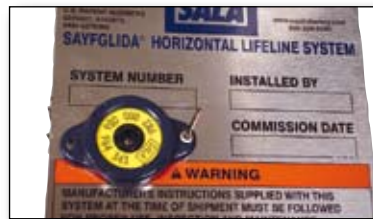
Cable Retrofit Tag Installation
